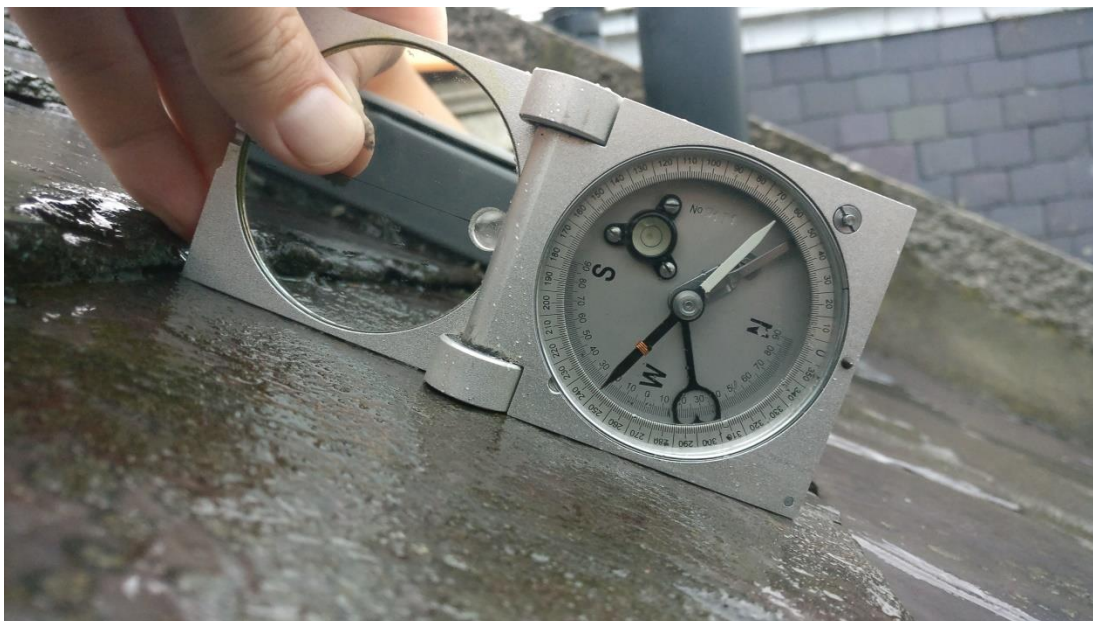
EXISTING ROOF to DWELLING indicating a roof pitch of 27.5 degrees.
